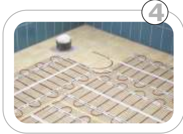
Ready to install tiles
